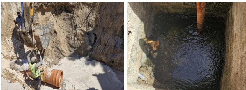
Figure 10: Dewatering well and Line in Zliten (Higher Technical Committee for Monitoring the Groundwater Overflow Phenomenon page, 2026).
