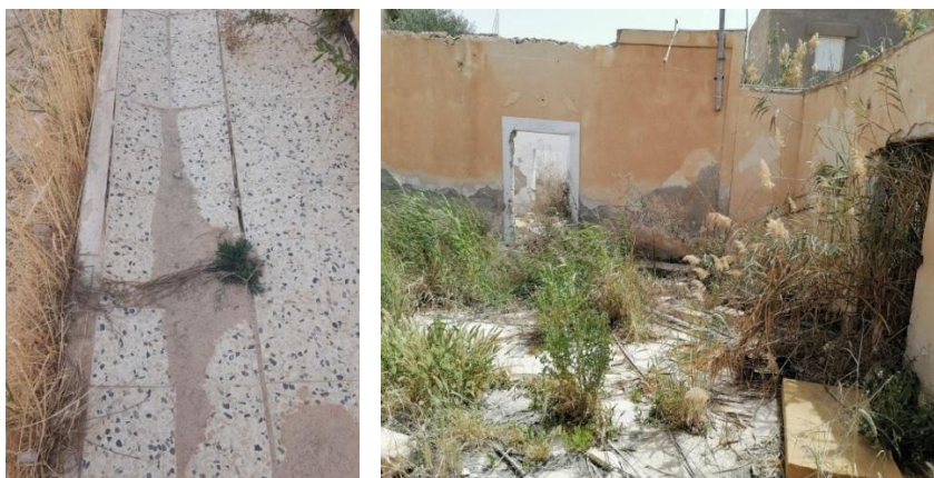
Figure 7: Ground Subsidence (Left) and Rising Dampness (Right), Resulting in the Abandonment of Several Residential Buildings.
